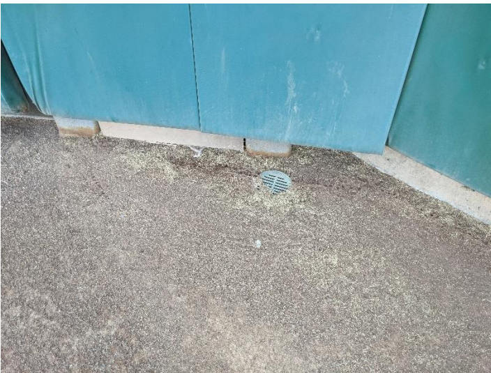
SECTION 7 (PLAYING FIELD) SURFACE DRAINS INSTALLED ON WARNING TRACK ARE NOT LEVEL WITH WARNING TRACK
